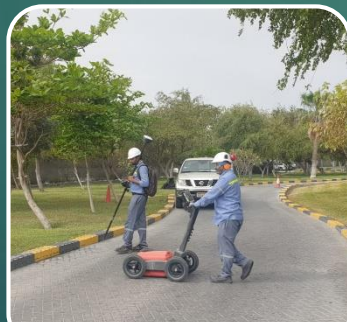
Execute the GPR work
